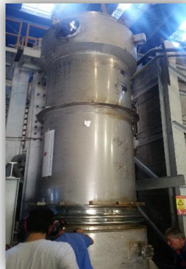
Recuperator installation
